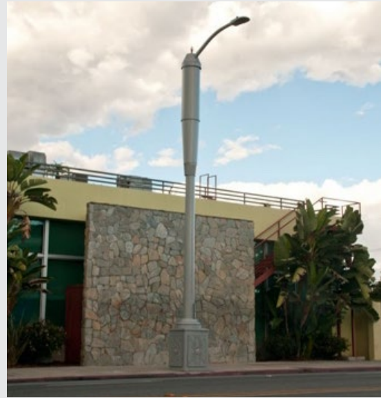
Figure 23 – City of Los Angeles street light and mobile phone transmission column (Philips / Ericsson)
